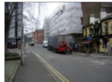
LOOKING SOUTH ALONG GREYFRIARS ROAD
