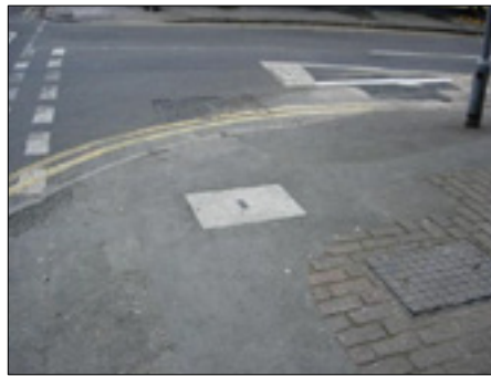
PHOTOGRAPH 5 VIRGIN MEDIA AND VODAFONE CHAMBERS AT JUNCTION OF GREYFRIARS ROAD WITH STANSHAW ROAD
