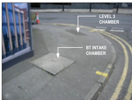
PHOTOGRAPH 1 EXISTING BT AND LEVEL 3 CHAMBERS OUTSIDE ENTRANCE AT JUNCTION OF VACHEL ROAD WITH GREYFRIARS ROAD
